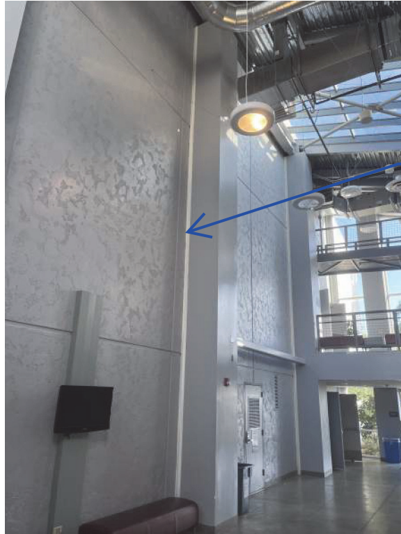
Seismic Separation @ 0007
