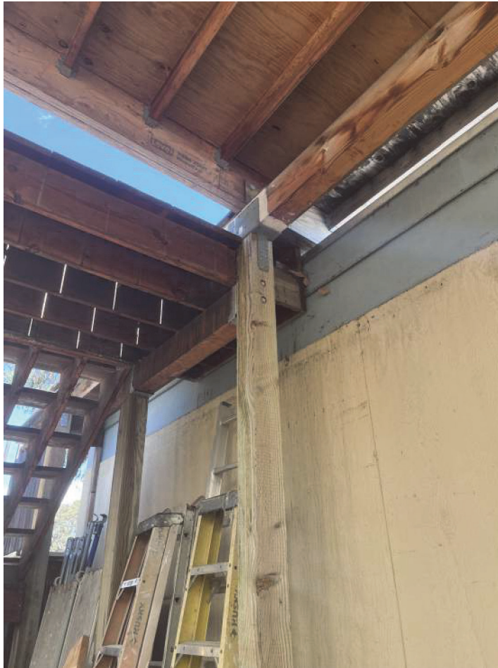
Stair, Landing, & High Roof Addition @ West Courtyard
