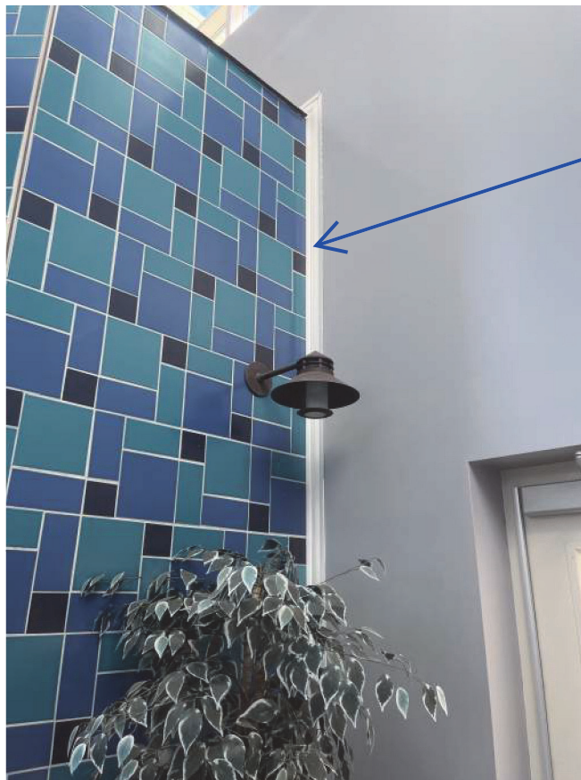
Seismic Separation @ 0007
