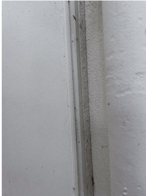
Seismic Separation @ Storage
