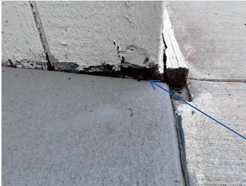
Pressure Treated Wood Sill-On-Ground
