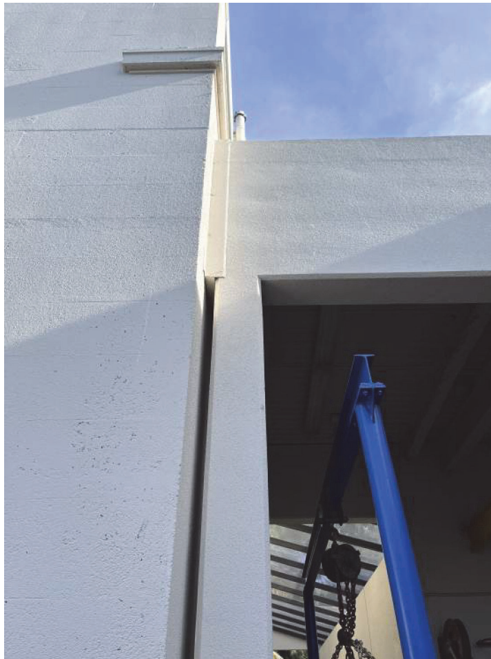
Seismic Separation @ 0001.1
