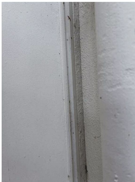
Seismic Separation @ Storage
