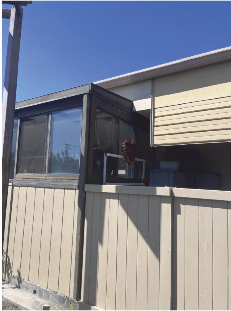
Addition @ South-West Corner - Exterior
