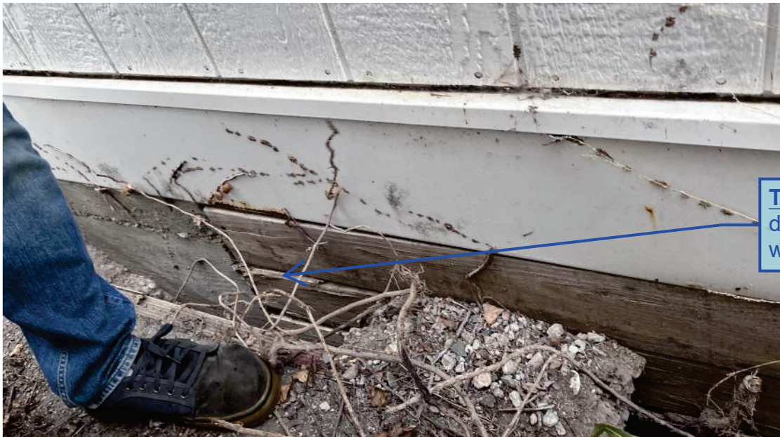
Wood Blockout for Sewage Drainage
