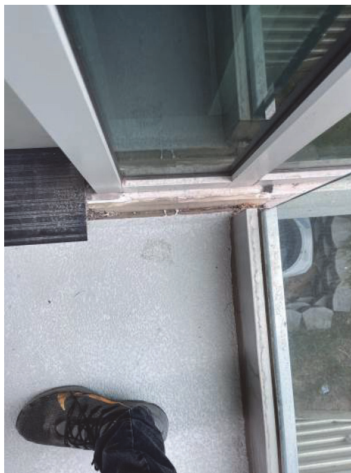
Seismic Separation @ Stair
