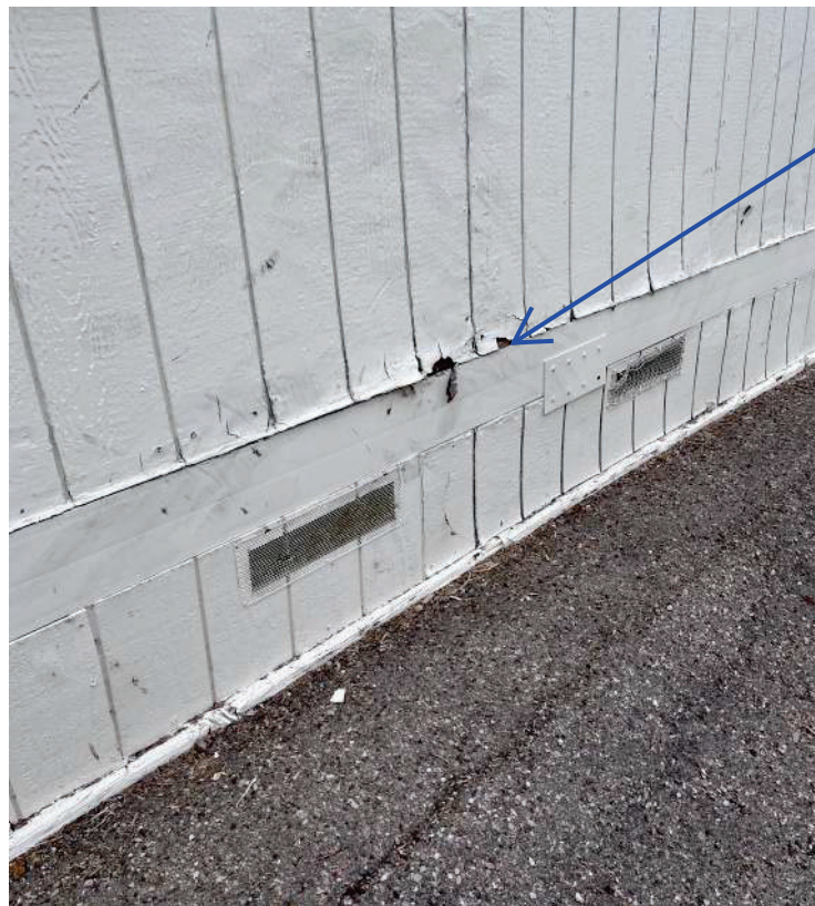
Wall Framing to Floor Framing Joint
