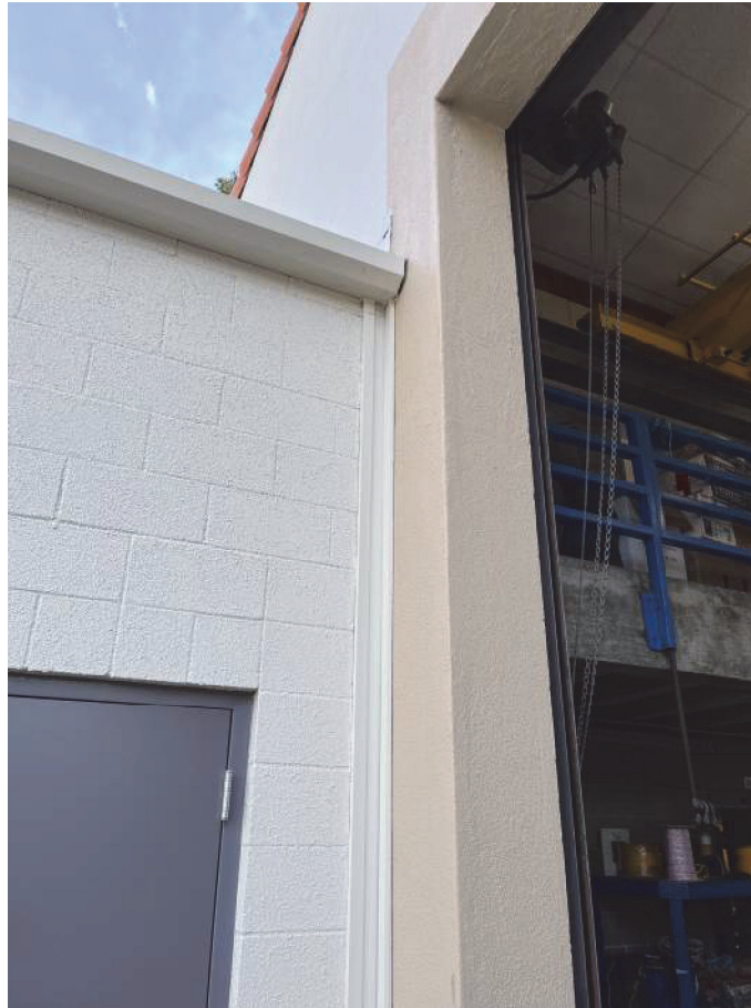
Seismic Separation @ 0016
